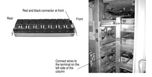
Check all battery connections to ensure that contact is established.
