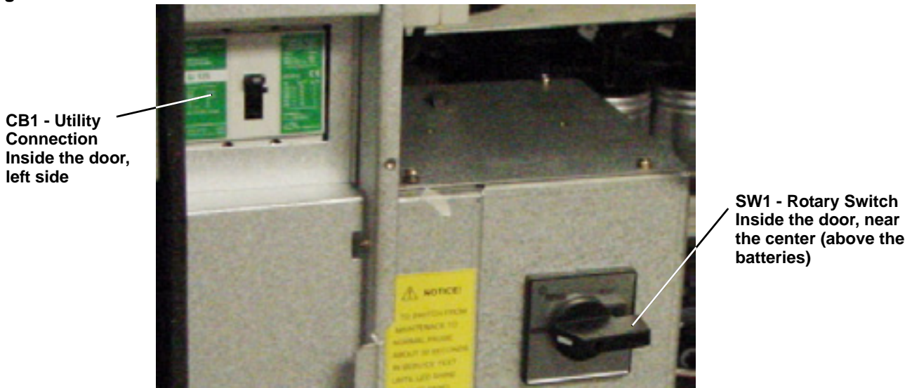
Figure 58 Power switches - 10kVA NX
